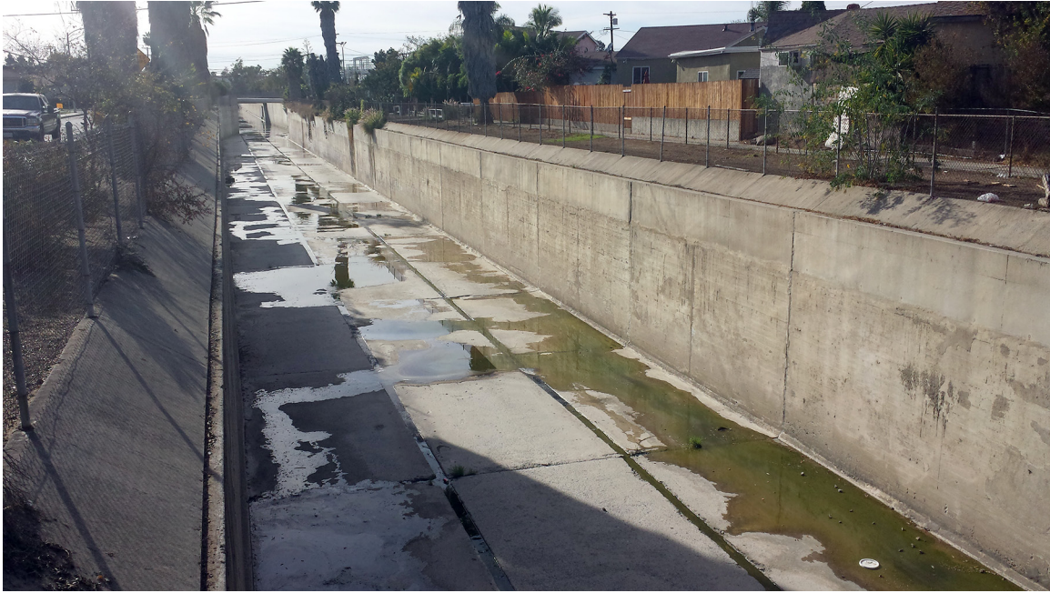
Typical concrete-lined Ballona Creek segment near Culver City.
