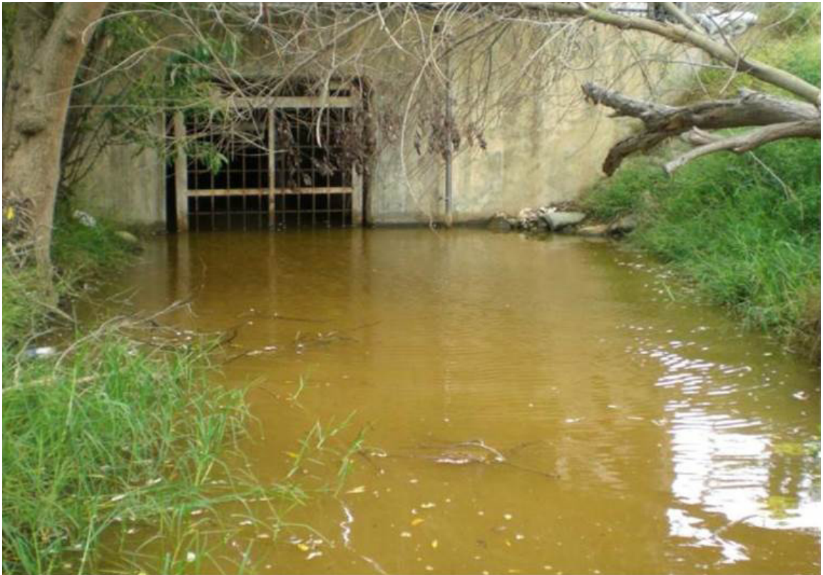
Drainage at Marie Canyon Low-Flow Diversion.
